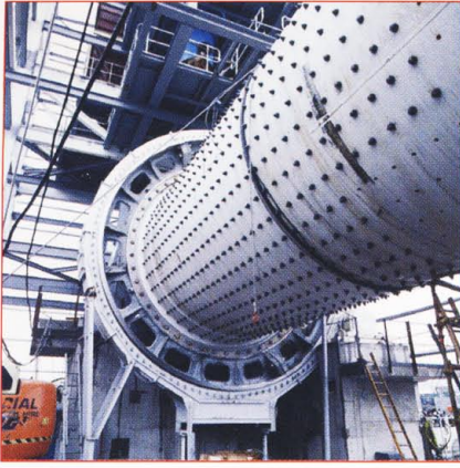
Online condition monitoring avoids unplanned downtimes of tube mills.
